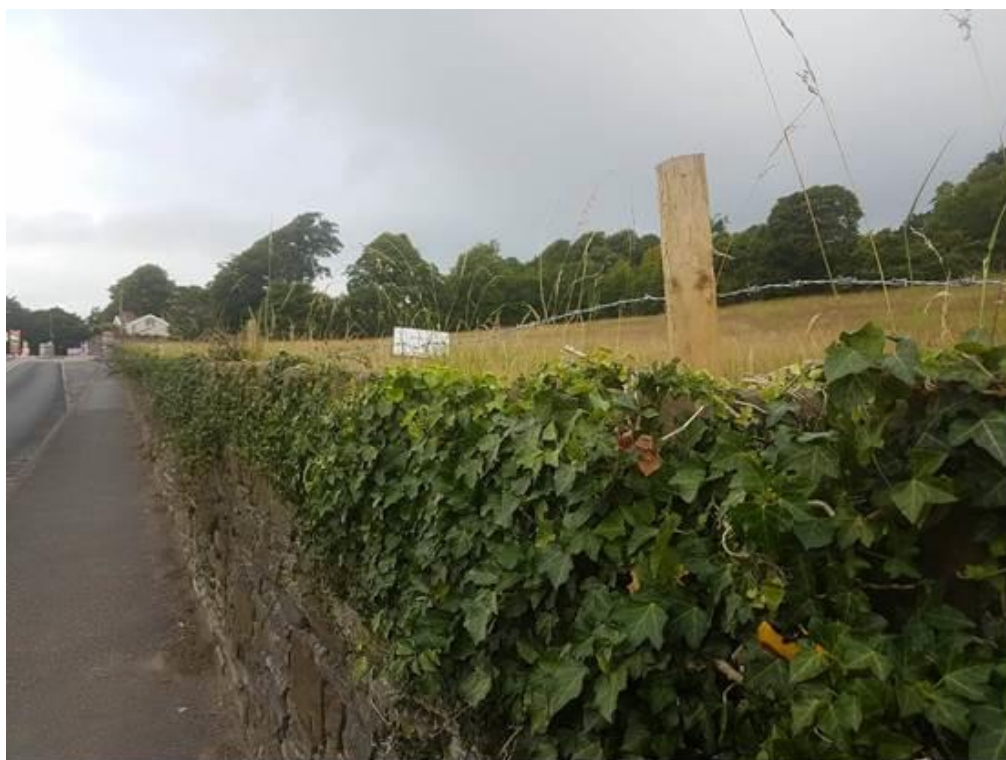
Plate 2 – Southern boundary (wall)
